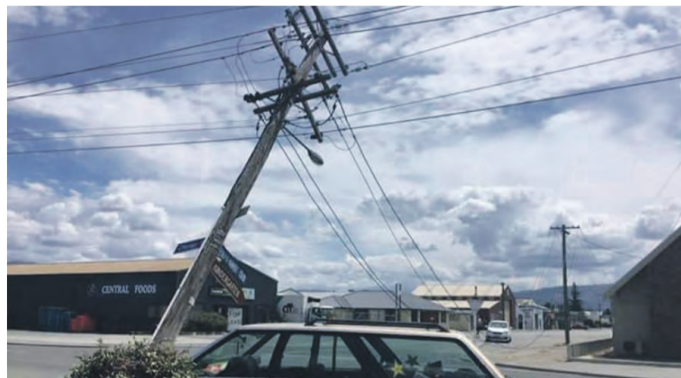
Many homes have not had power reconnected.
